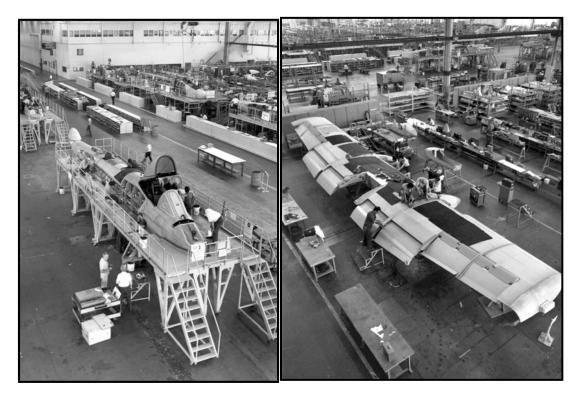
Figure 19. A-10 Fuselage and Wing Production<sup>10</sup>
